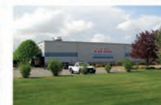
UST Chicopee Plant
